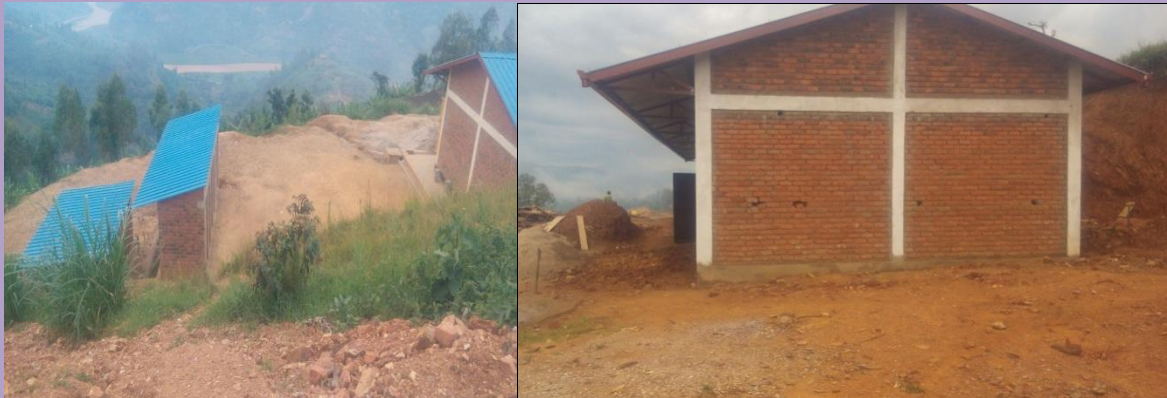
Gisura Primary school 3 classrooms were built at Ngaru Parish.
