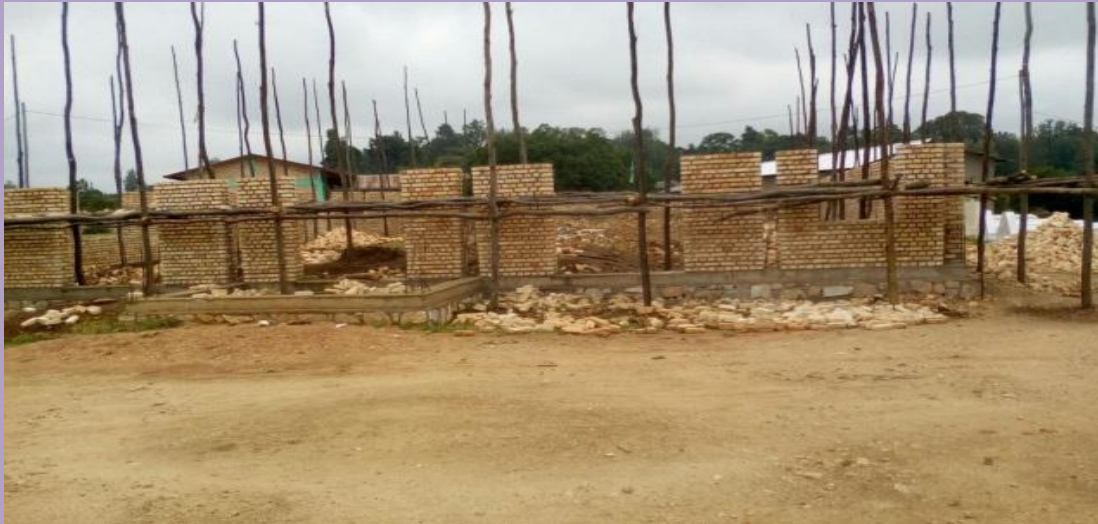
Construction of church building at Hanika Parish
