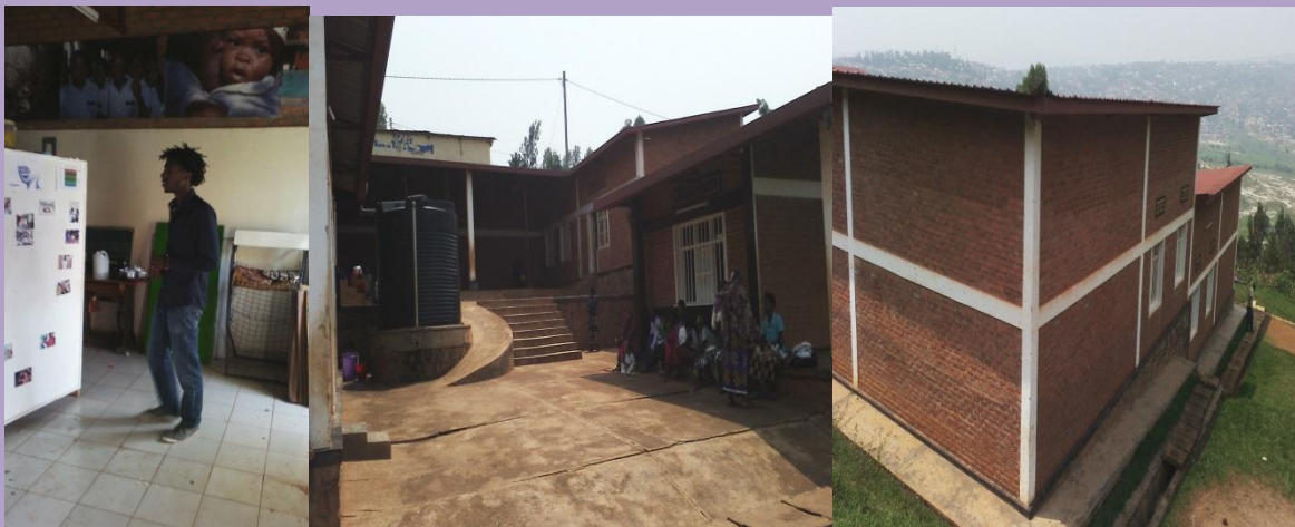
Root Foundation where Mr. Lucas is working
