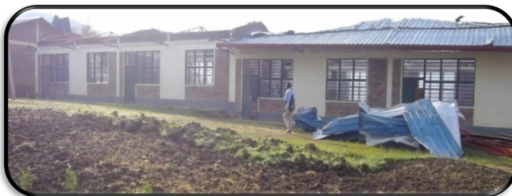
Figure 17: Shaki School was destroyed by the wind
