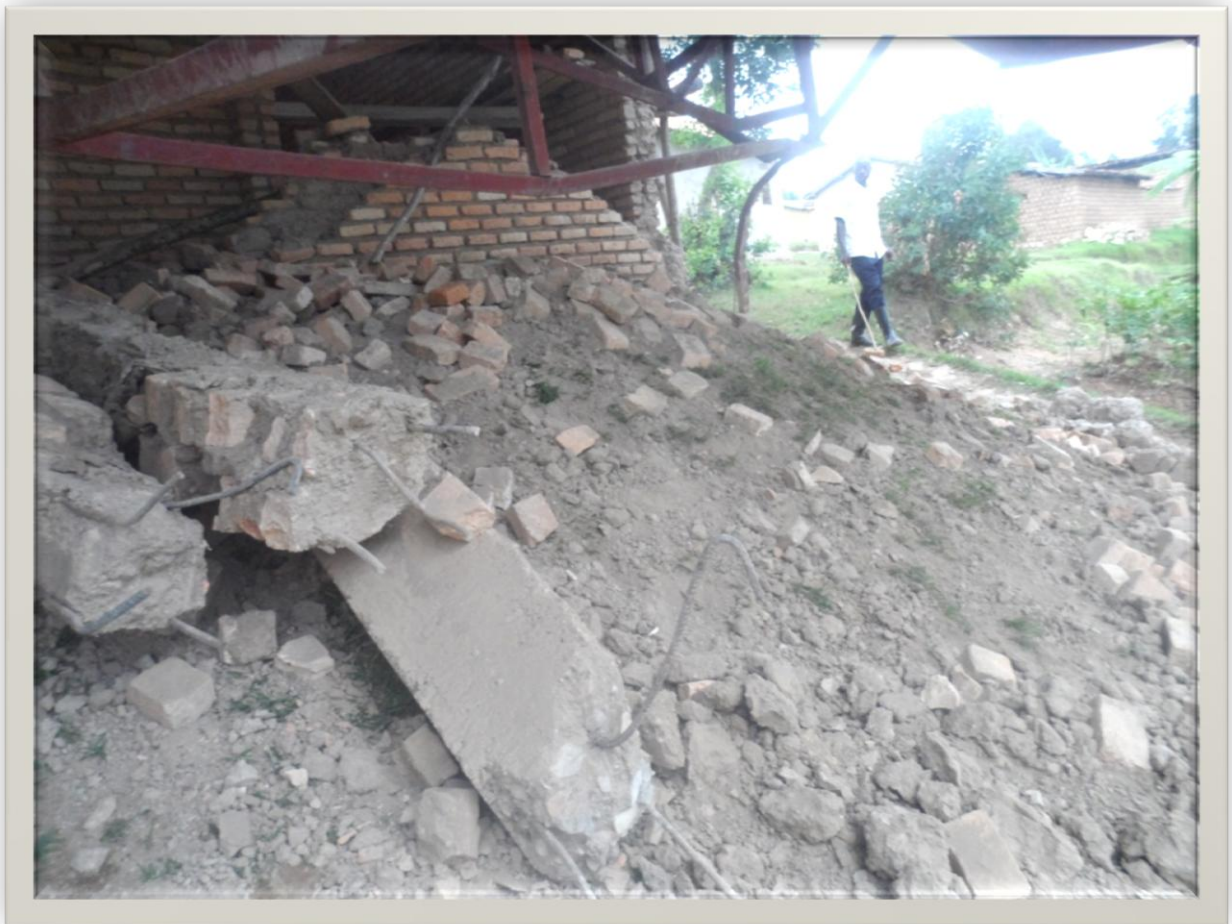
Figure 3: Gikomero church building has fallen down
